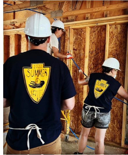
David, Fin & Vicky installing those water lines
