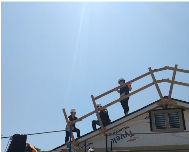
Nikki and Diana taking down scaffolding
