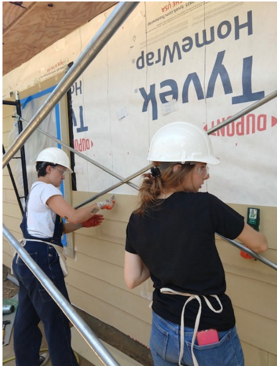
Janelle and Heather installing siding
