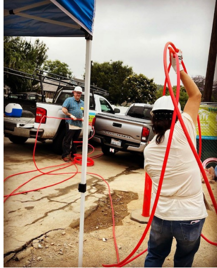
Aaron and Vicky unraveling water lines
