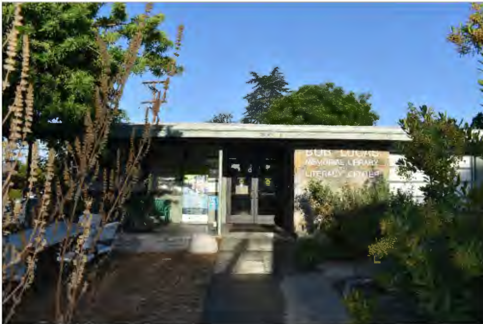
East elevation, facing west.
