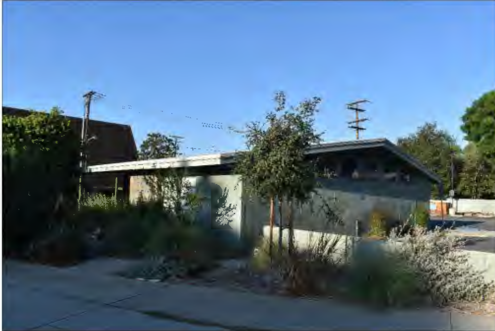
North and east elevations, facing southwest.
