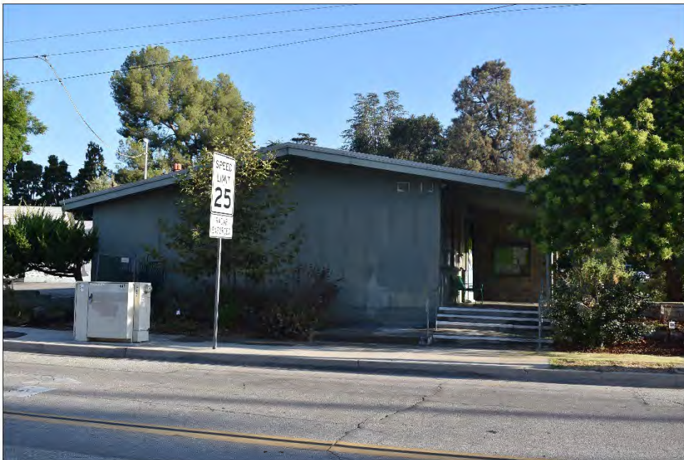
South elevation, facing north.
