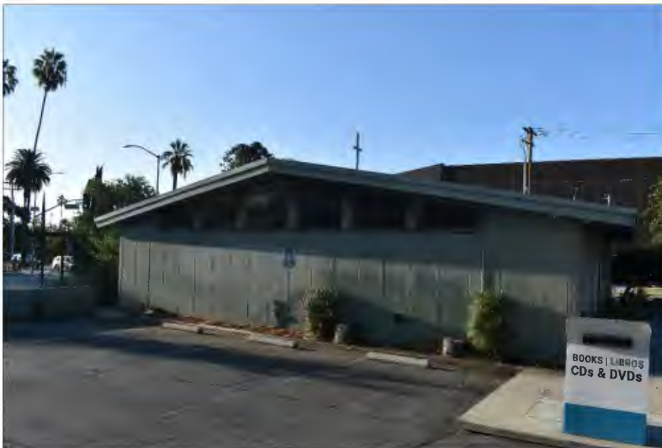
North elevation, facing south.
