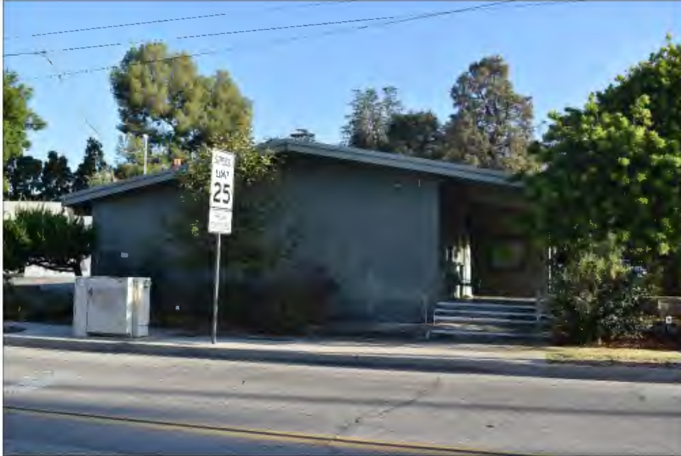
South elevation, facing north.
