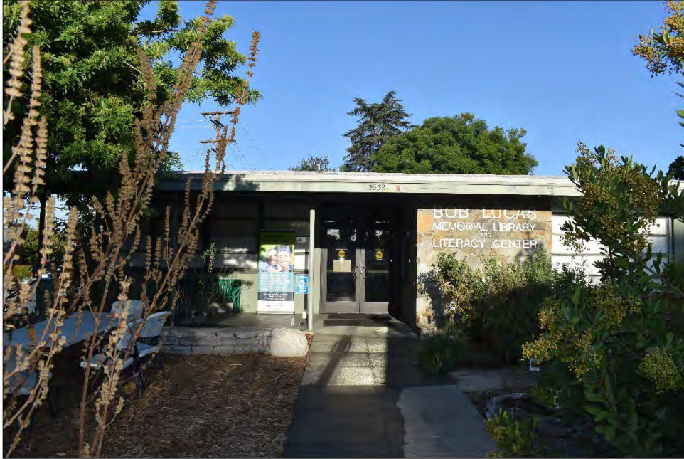
East elevation, facing west.
