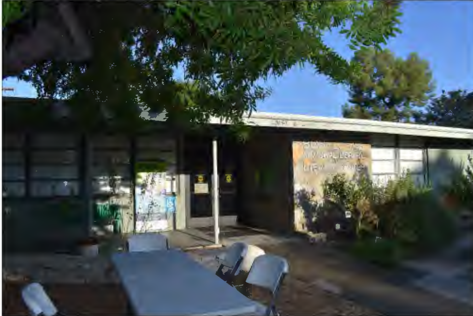
East elevation, facing northwest.
