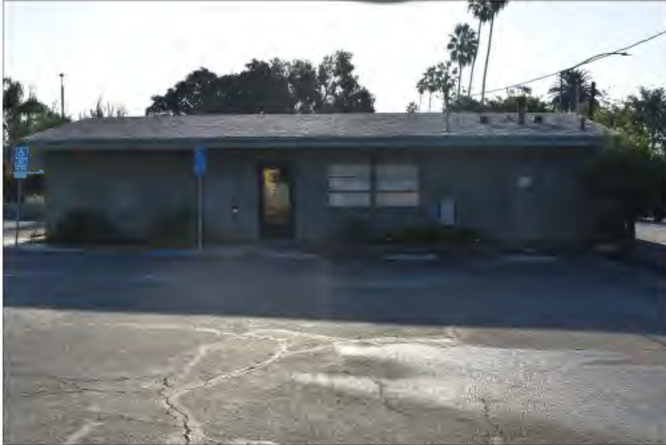
West elevation, facing east.
