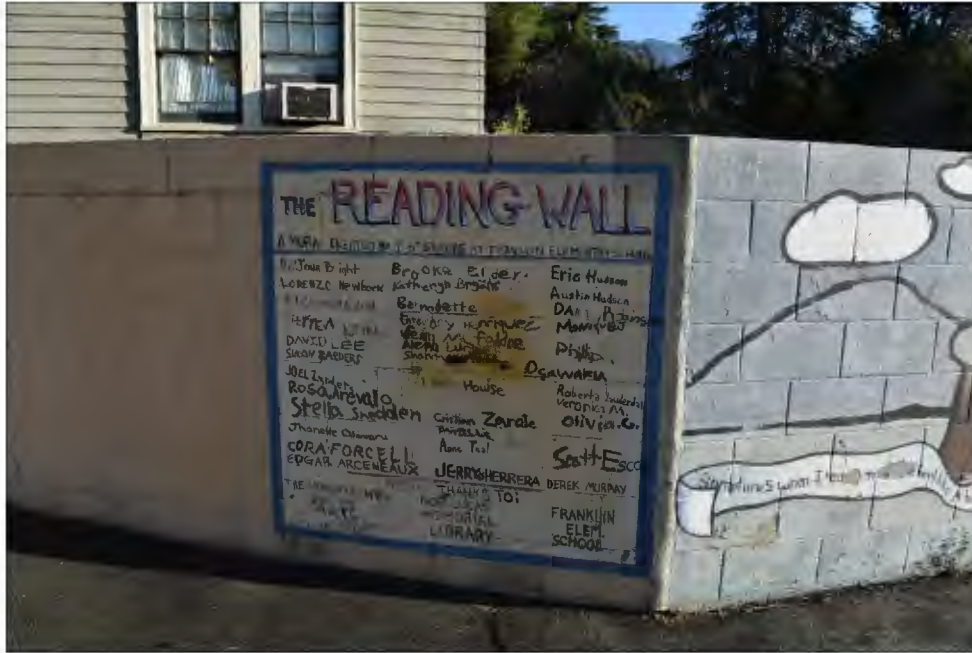
Mural wall detail, facing north.
