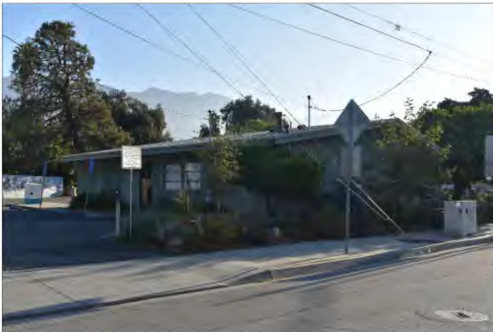
South and west elevations, facing northeast.
