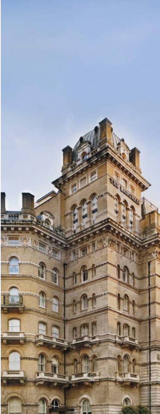
Langham Hotel Historical Renovation, London
