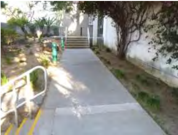
0001026a 4/24/2018 Concrete sidewalk settlement repairs Southeast sidewalk to south entrance
