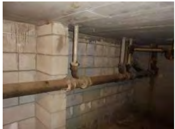
0001088e 4/24/2018 Original drain piping First floor, crawlspace
