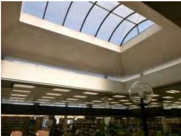
0001052a 4/24/2018 Elliptical skylight and painted and suspended grid ceilings Second floor, library, over sunken area
