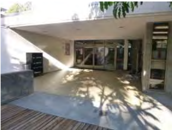
0001015a 4/24/2018 Sliding glass entrance doors and tile entrance Main entrance to library, east side
