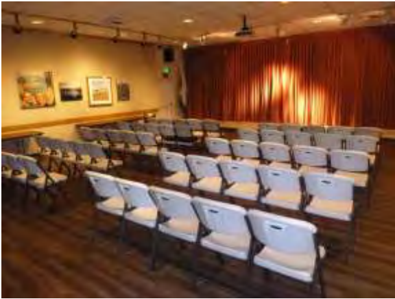
0001055a 4/24/2018 Laminate floor, suspended grid ceiling tile, wallpaper, and LED exit Split-level conference room, east side
