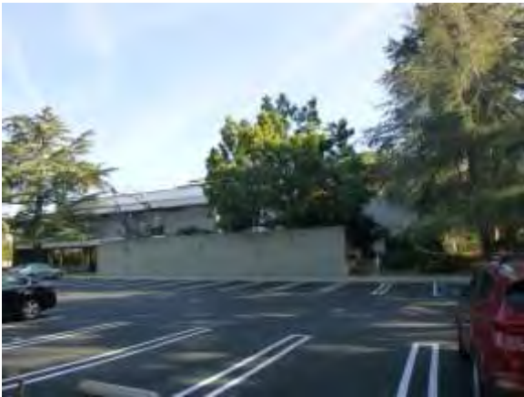
0001023a 4/24/2018 South elevation South side of building
