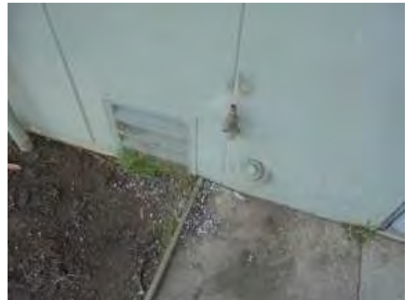
0002009e 4/24/2018 Original drain clean out Building exterior
