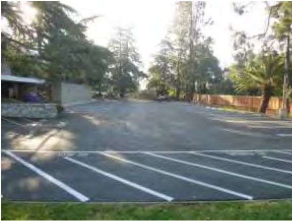
0001001a 4/24/2018 Recently repaved and sealcoated asphalt parking lot South side parking looking east
