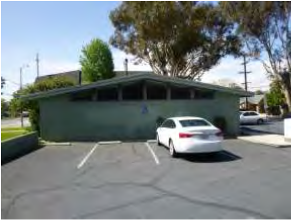
0002001a 4/24/2018 North elevation, asphalt pavement, and painted concrete wall North side of building
