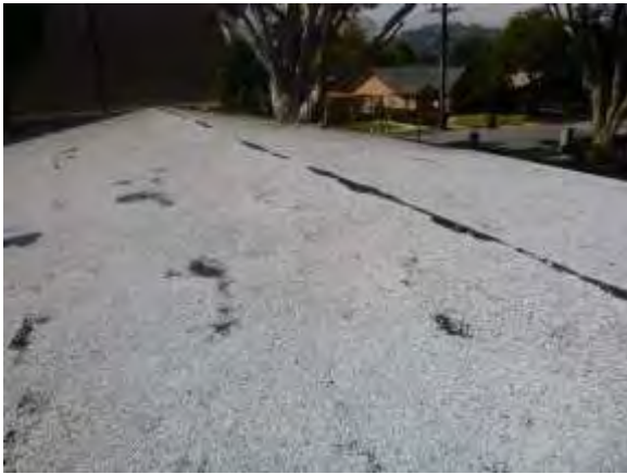
0002008a 4/24/2018 Sloped built-up roof with pea gravel ballast Roof, looking south
