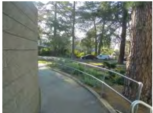
0001012e 4/24/2018 Lack of exterior lighting Site
