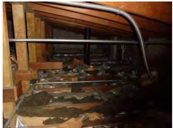
0002037e 4/24/2018 Blown in insulation Attic
