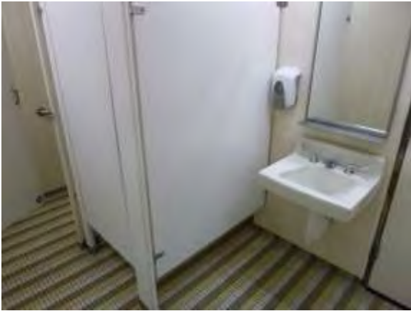
0001058a 4/24/2018 Ceramic tile floor and walls and old sink and partition Split-level women's restroom
