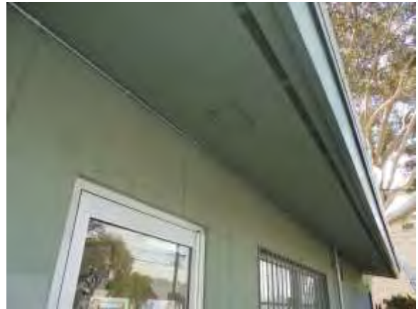
0002017e 4/24/2018 Exterior lighting Building exterior
