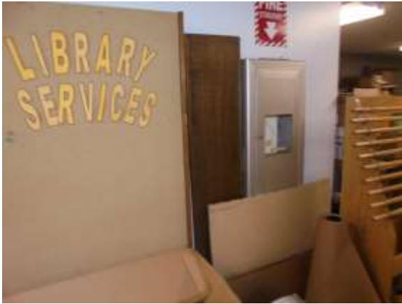
0001095e 4/24/2018 Fire extinguisher in cabinet First floor, corridor
