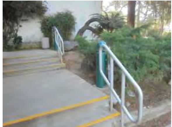
0001019e 4/24/2018 Exterior lighting Site
