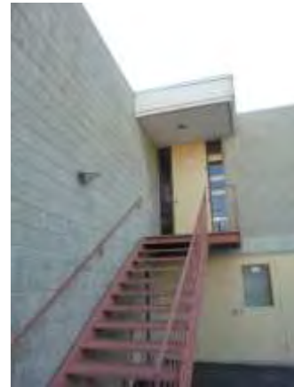
0001002e 4/24/2018 Exterior lighting Building exterior
