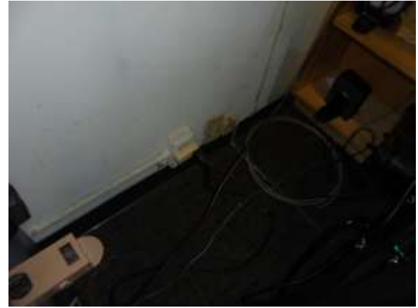
0002041e 4/24/2018 Electrical outlet Staff room
