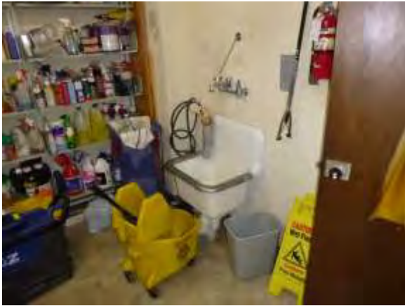
0001067a 4/24/2018 Service sink, roll vinyl floor, and knob door hardware First floor, custodial closet
