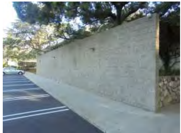
0001018e 4/24/2018 Exterior lighting Building exterior
