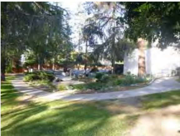
0001018a 4/24/2018 Landscaping, sidewalk, missing handrails, and protected trees East-southeast side of building
