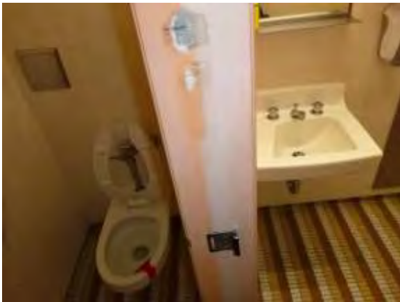
0001072a 4/24/2018 Old restroom fixtures and ceramic tile floor and walls First floor, men's restroom
