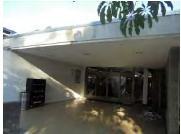
0001008e 4/24/2018 Exterior lighting Building exterior
