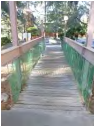
0001020a 4/24/2018 Damaged, rotted, uneven wood planks on pedestrian bridge Southeast side of facility
