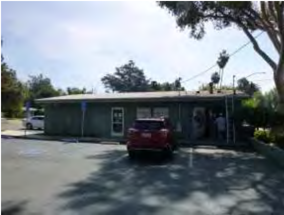
0002002a 4/24/2018 West elevation, handicap parking, and west entrance West side of building
