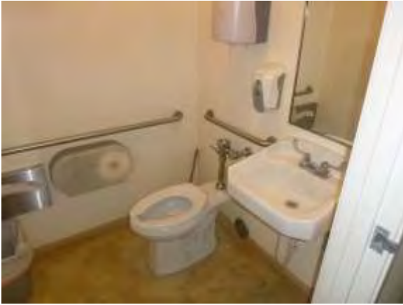
0002014a 4/24/2018 Restroom fixtures Restroom, typical
