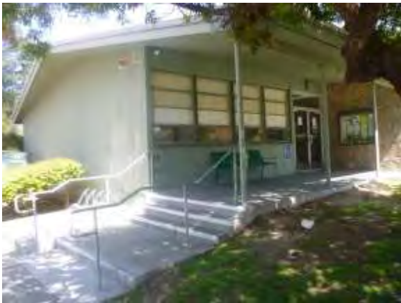
0002004a 4/24/2018 Compliant handrails, single-pane windows, and east entrance Southeast side of building
