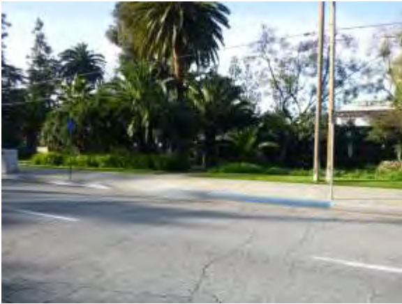
0001007a 4/24/2018 Designated curb side handicap parking and curb cut Mariposa Street, north side of facility
