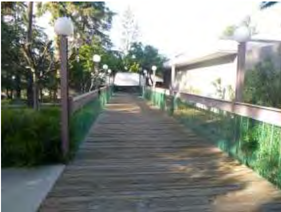
0001014a 4/24/2018 Steel and timber pedestrian bridge with uneven surface Access to library entrance, second level
