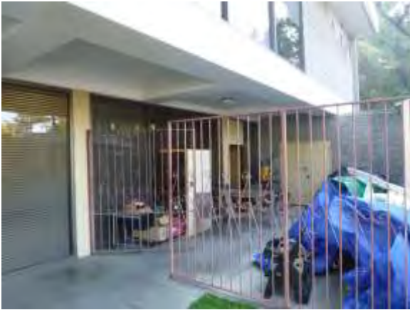
0001028a 4/24/2018 Storage area and metal doors First floor, south side
