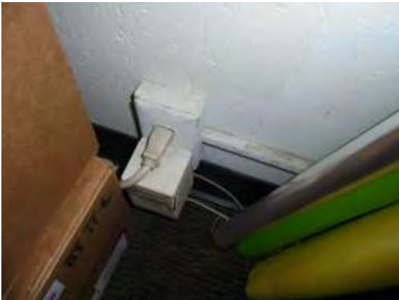
0002042e 4/24/2018 Electrical outlet Staff room
