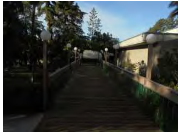
0001006e 4/24/2018 Exterior lighting Site
