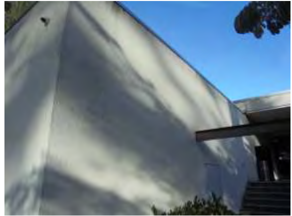
0001010e 4/24/2018 Lack of exterior lighting Building exterior
