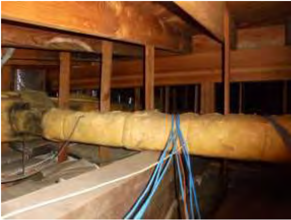
0002038e 4/24/2018 Duct insulation Attic
