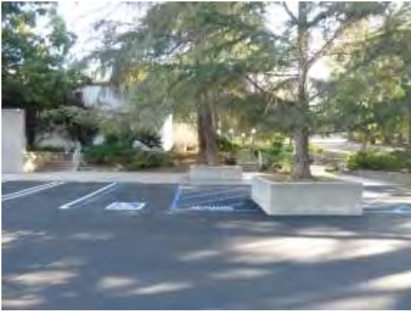
0001022a 4/24/2018 Designated handicap van parking South parking lot, east side
