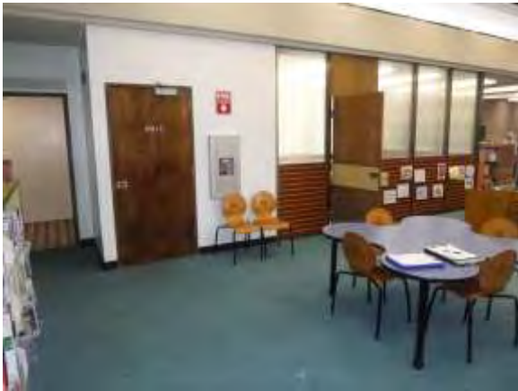
0001047a 4/24/2018 Old wood doors, knobs, missing Braille, and carpet squares Second floor, library, south side
