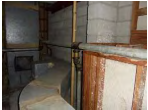
0001049e 4/24/2018 Original drain piping Second floor, attic area
