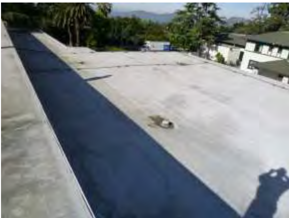
0001036a 4/24/2018 Roll asphalt roof Roof, west side looking south
