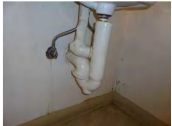
0002019e 4/24/2018 Supply and drain piping Men's restroom
