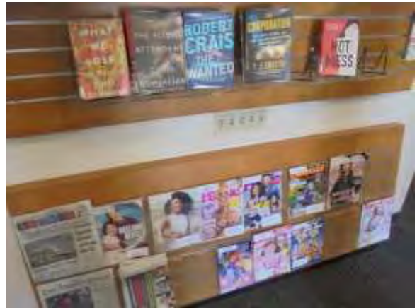
0002035e 4/24/2018 Electrical switches at low height Main room
