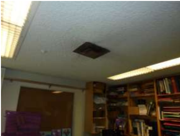
0002028e 4/24/2018 Interior lighting Staff room
