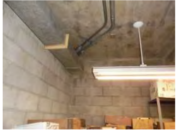
0001092e 4/24/2018 Original ductwork and interior lighting First floor, book storage room
