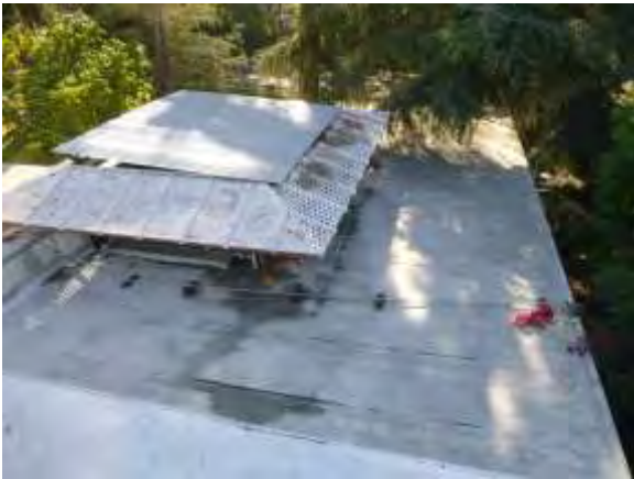
0001029a 4/24/2018 Roll asphalt roof, corrugated metal roof, and metal screens Roof over southeast conference room
