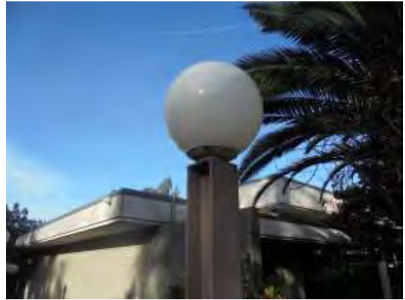
0001007e 4/24/2018 Exterior lighting Site
