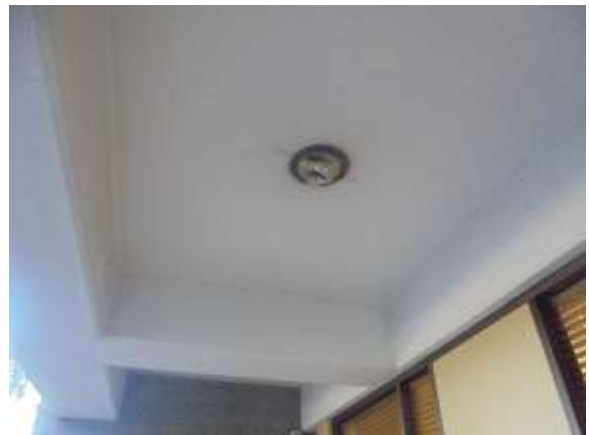
0001024e 4/24/2018 Exterior lighting Building exterior
