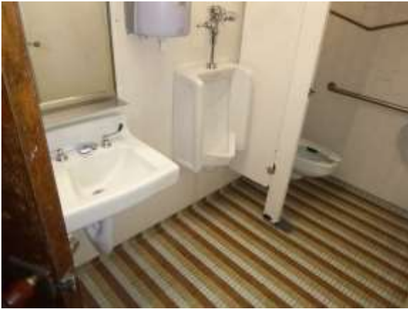
0001049a 4/24/2018 Restroom fixtures and finishes, door that opens in, and knob hardware Second floor, men's restroom
