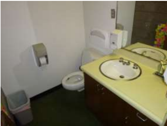
0001044a 4/24/2018 Countertop sink and low flow toilet with tank Second floor, director's office bathroom
