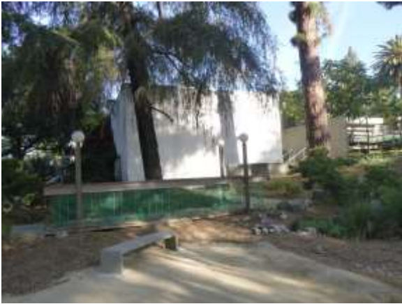
0001019a 4/24/2018 Pedestrian bridge and landscaping Southeast side of facility
