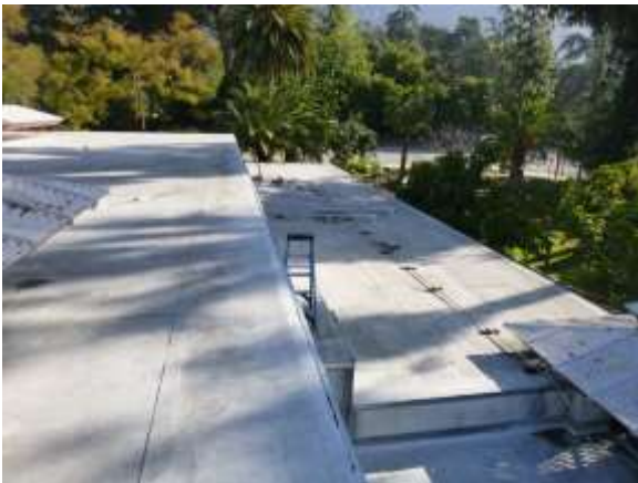
0001030a 4/24/2018 Roll asphalt roofs Roof, east side looking north
