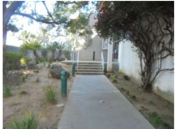
0001020e 4/24/2018 Exterior lighting Site
