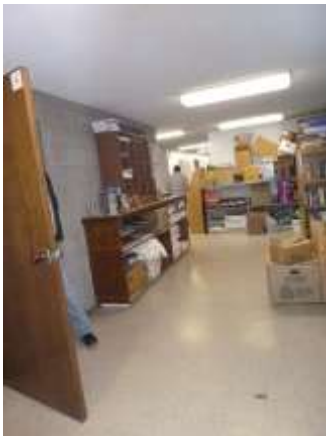
0001063a 4/24/2018 9-inch square floor tile, painted ceilings, and knob hardware First floor, hallway
