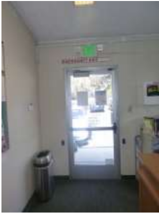
0002016a 4/24/2018 LED exit sign and lack of door operator West side entrance/exit
