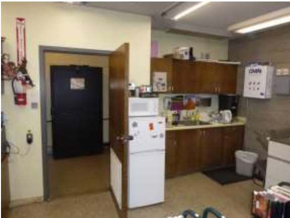
0001039a 4/24/2018 Old cabinets, knob door hardware, and 9- and 12-inch tile Second floor, east side rooms
