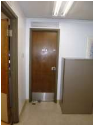
0001071a 4/24/2018 Narrow restroom entrance door, knob hardware, and lack of Braille First floor, hallway
