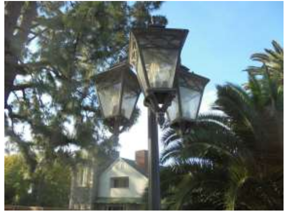
0001025e 4/24/2018 Exterior lighting Site
