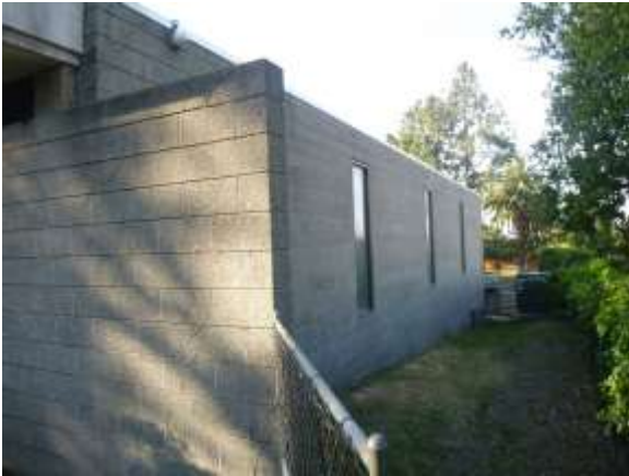
0001005a 4/24/2018 Northwest elevation, windows, and CMU exterior West-northwest side of building
