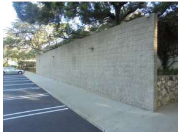
0001018e 4/24/2018 Exterior lighting Building exterior
