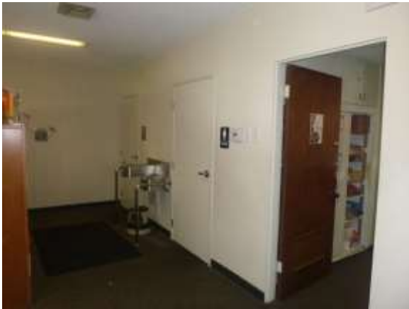
0002011a 4/24/2018 Dual-level fountain, restroom entrances, and knob door hardware Library interior, southwest side
