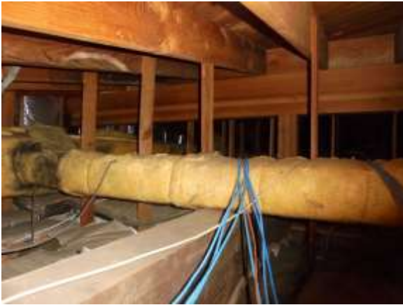
0002038e 4/24/2018 Duct insulation Attic
