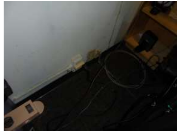
0002041e 4/24/2018 Electrical outlet Staff room
