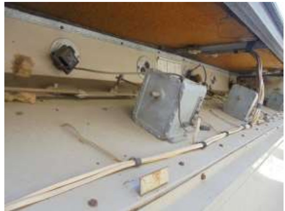
0001030e 4/24/2018 Damper section of rooftop package unit #1 Roof
