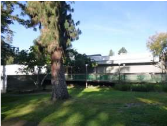
0001017a 4/24/2018 Northeast elevation and CMU and stucco siding Northeast side of building
