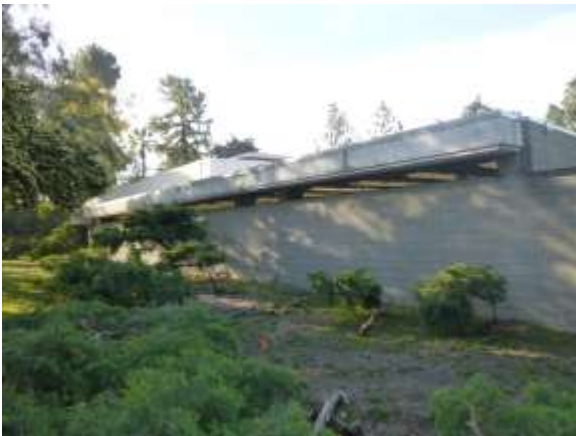
0001006a 4/24/2018 North-northwest elevation and landscaping Northwest side of building
