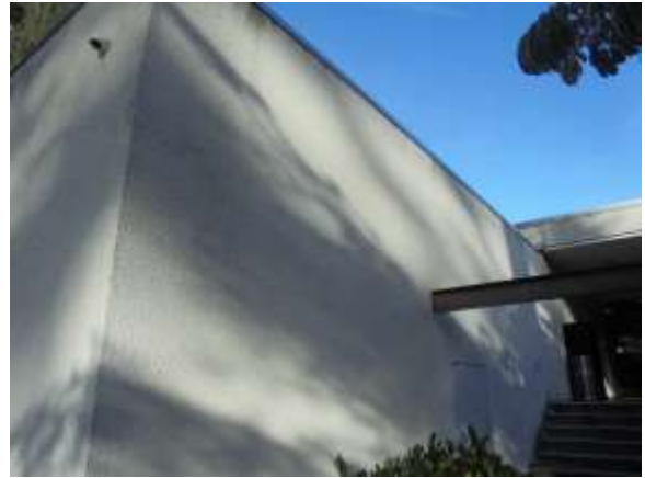
0001010e 4/24/2018 Lack of exterior lighting Building exterior
