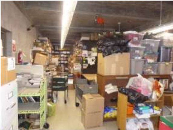
0001064a 4/24/2018 9-inch vinyl floor and open structural concrete ceiling First floor, storage room
