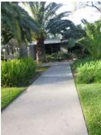
0001009a 4/24/2018 Concrete sidewalk repair, lack of handrails, and landscaping North side access from curb cut
