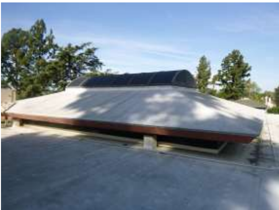
0001033a 4/24/2018 Skylight Central roof
