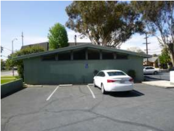
0002001a 4/24/2018 North elevation, asphalt pavement, and painted concrete wall North side of building
