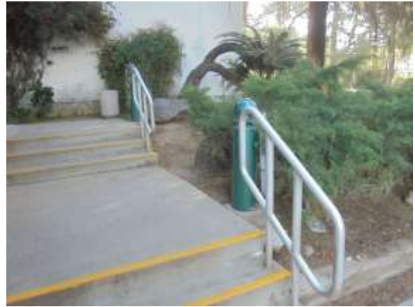
0001019e 4/24/2018 Exterior lighting Site
