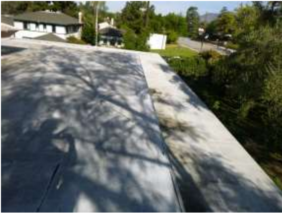
0001034a 4/24/2018 Roll asphalt roof with exposed seam Roof, north side looking west
