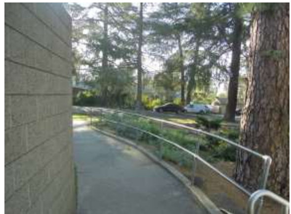
0001012e 4/24/2018 Lack of exterior lighting Site
