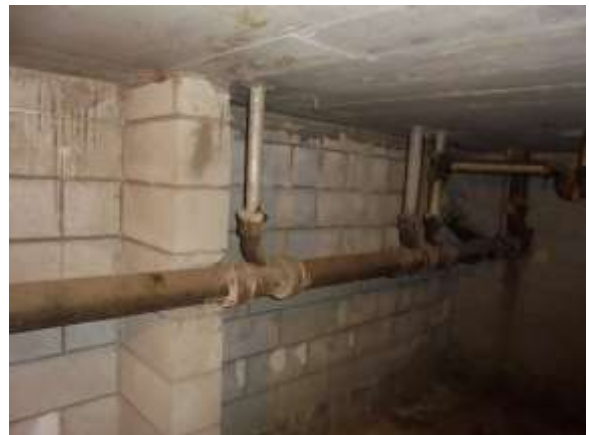
0001088e 4/24/2018 Original drain piping First floor, crawlspace
