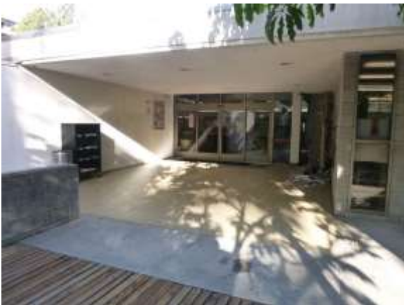
0001015a 4/24/2018 Sliding glass entrance doors and tile entrance Main entrance to library, east side
