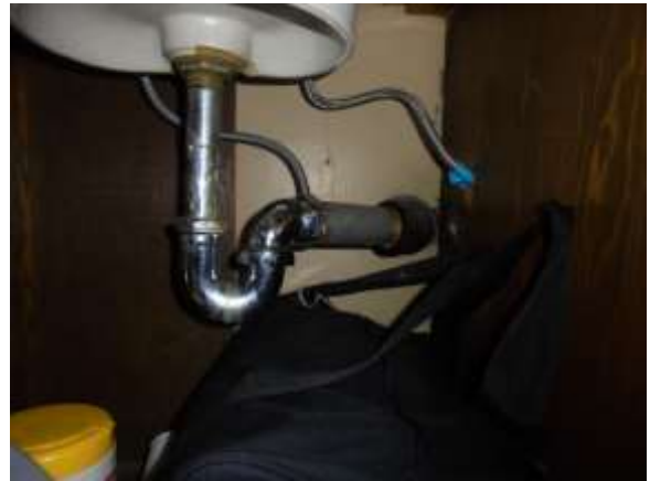
0001071e 4/24/2018 Supply and drain piping Second floor, director's office, restroom
