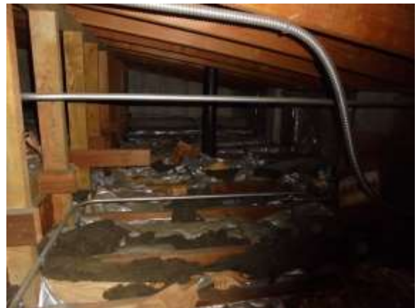
0002037e 4/24/2018 Blown in insulation Attic
