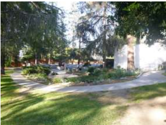
0001018a 4/24/2018 Landscaping, sidewalk, missing handrails, and protected trees East-southeast side of building
