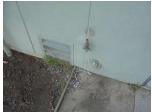
0002009e 4/24/2018 Original drain clean out Building exterior
