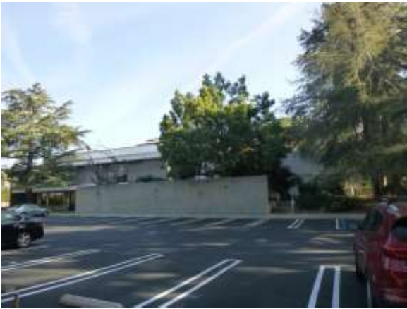
0001023a 4/24/2018 South elevation South side of building
