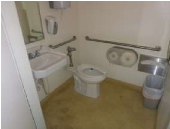
0002013a 4/24/2018 Remodeled accessible restroom with ceramic tile floor Restroom, typical
