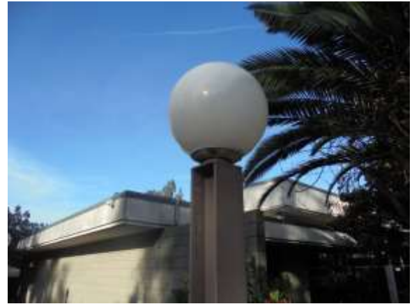
0001007e 4/24/2018 Exterior lighting Site
