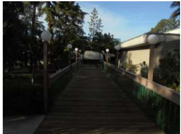
0001006e 4/24/2018 Exterior lighting Site
