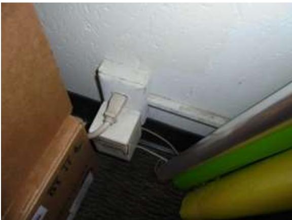
0002042e 4/24/2018 Electrical outlet Staff room
