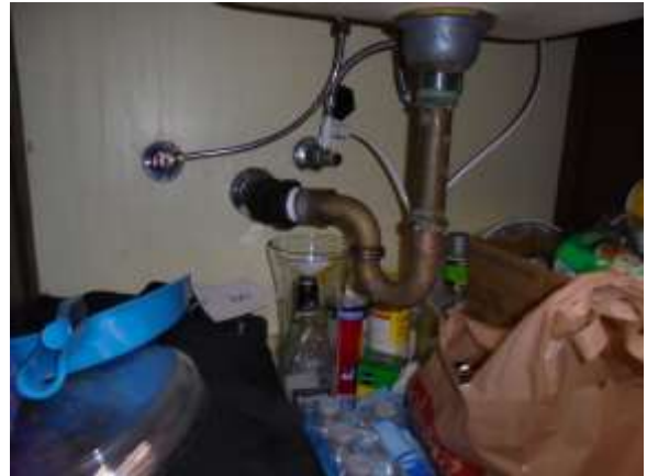
0001043e 4/24/2018 Supply and drain piping Second floor, circulation room
