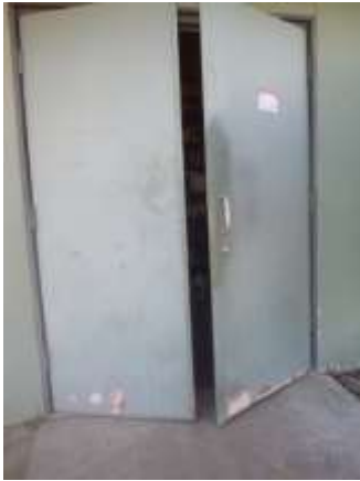
0002007a 4/24/2018 Mechanical room doors that are delaminated at the bottom Mechanical room, southwest side of building
