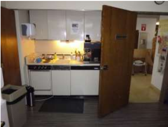
0001065a 4/24/2018 Old kitchenette, laminate flooring, and knob door hardware First floor, breakroom
