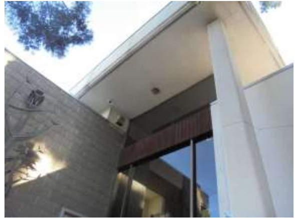
0001022e 4/24/2018 Exterior lighting Building exterior
