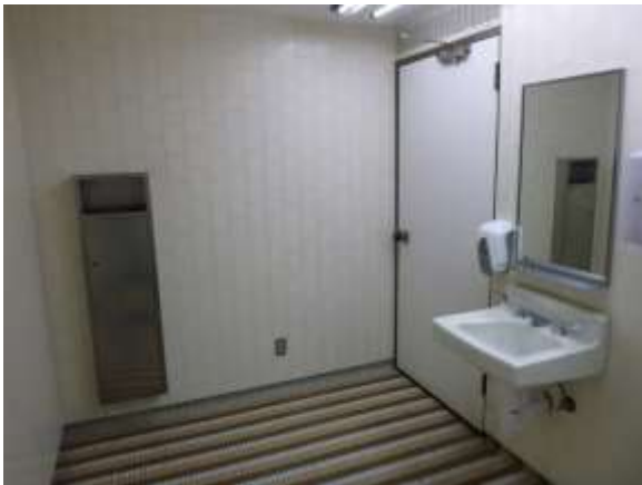
0001061a 4/24/2018 Entrance door Split-level men's restroom
