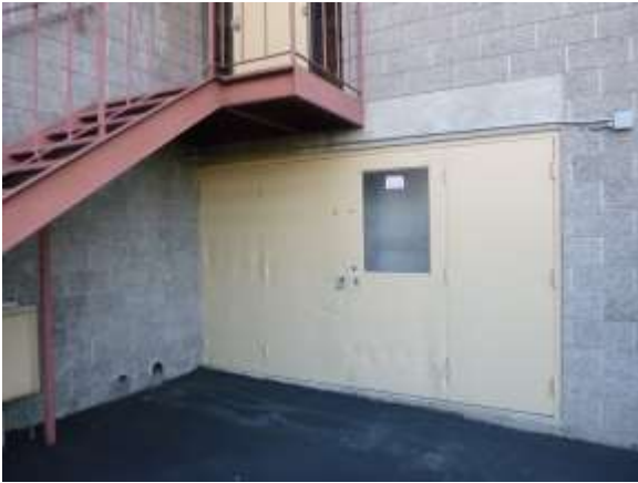
0001004a 4/24/2018 Old metal doors to electrical and mechanical area and CMU exterior First floor, west side
