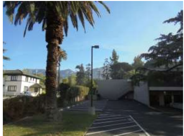
0001026e 4/24/2018 Exterior lighting Site
