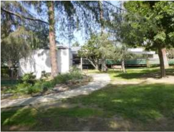
0001073a 4/24/2018 East elevation and missing sidewalk handrails East side of facility
