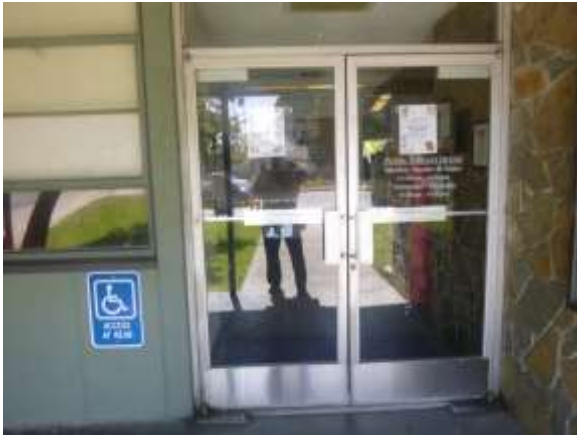
0002010a 4/24/2018 Old metal-framed glass entrance doors and hardware East entrance
