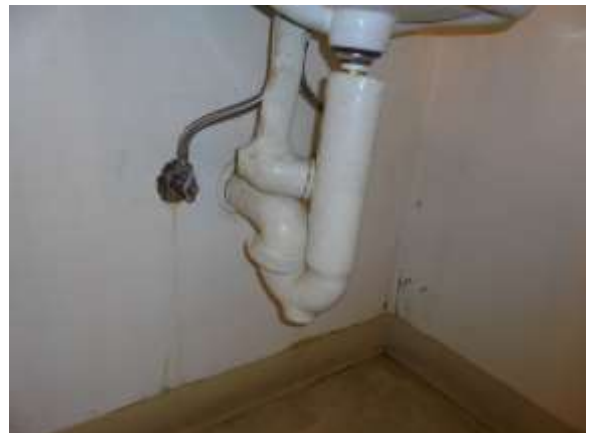
0002019e 4/24/2018 Supply and drain piping Men's restroom
