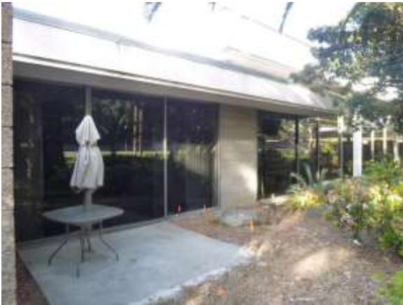
0001011a 4/24/2018 Patio, sliding glass window, and CMU and stucco exterior Northeast side of building
