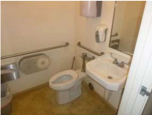
0002014a 4/24/2018 Restroom fixtures Restroom, typical
